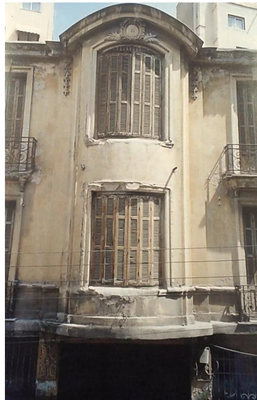
Picture 3: Detail of the front view
